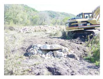
Fig. 8. Construction of a hibernaculum as part of a stream restoration project.
