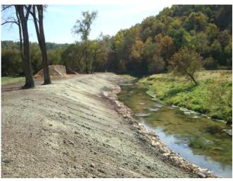
Fig. 11. Vertical nesting bank in background. Note its location set back from the stream channel.
