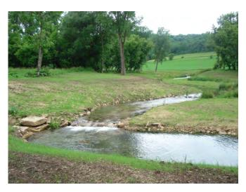
Fig. 1. Restored Driftless Area stream with armoring of the bank toe. Credit: Dauwal-
