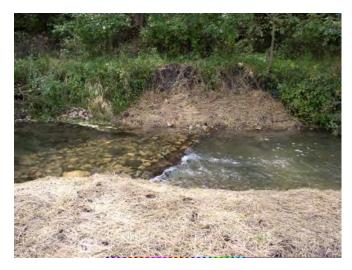
Fig. 13. Crosslog used to create pool habitat as part of a stream restoration project.
