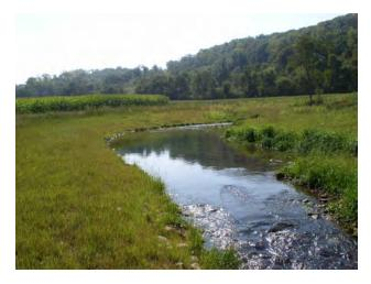
Fig. 4. Recently restored Driftless Area stream with stream buffer, sloped banks, and armored streabank toe.
