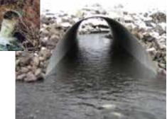
Culverts (above left) prevented fish from freely moving from Maggie Creek into Beaver Creek, a major tributary. In 2005 they were replaced with this fish-friendly structure (above) to connect the streams.
